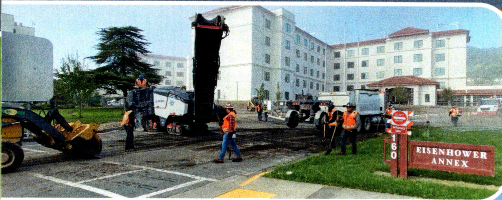
Above: Performing digout repairs on main drive isle of the existing main road of the Veterans Home facility.
