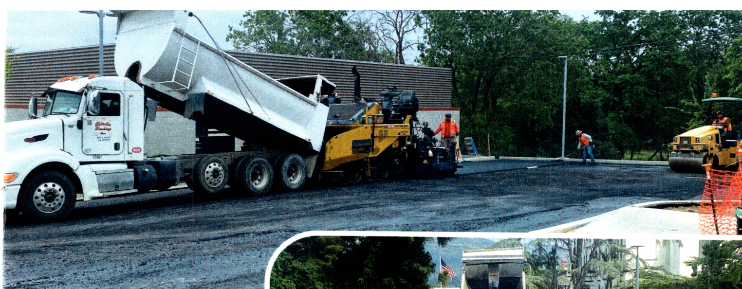
Above: McGuire & Hester using their Cat 1055F paver to place the first lift for the drive aisle to the central utility plant of the new skilled nursing facility in Napa Valley.
